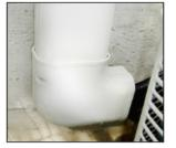
All penetrations through the shell of the home must be sealed with insulative sealant, any insulation disturbed by installed line set must be returned to original (or better) condition
