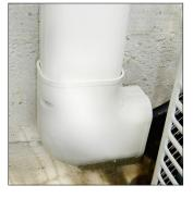
All penetrations through the shell of the home must be sealed with insulative sealant, any insulation disturbed by installed line set must be returned to original (or better) condition
